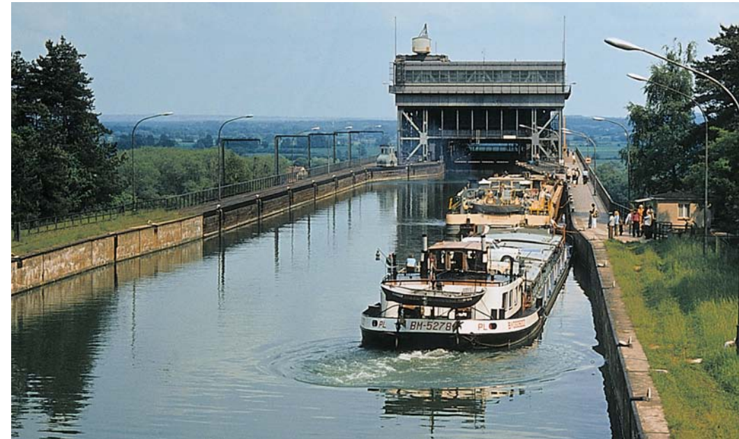
View of the boat lift from the west
