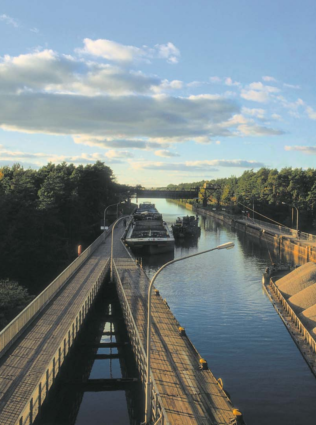
A ship arrives in the caisson of the boat lift from the upper approach
