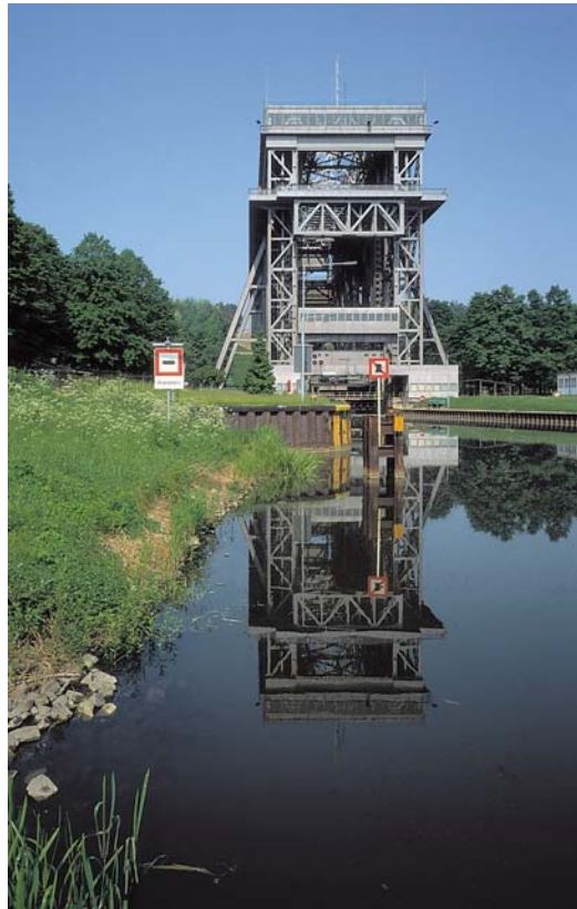
View of the boat lift from the south of the lower approach
