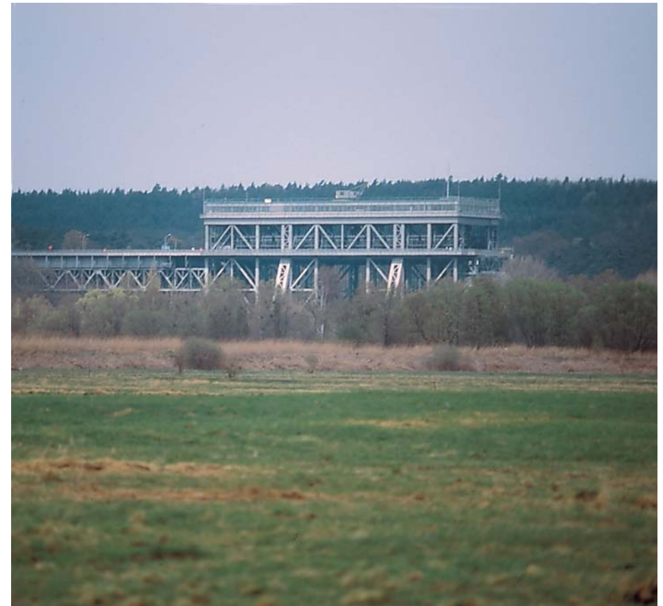
View of the boat lift from the south
